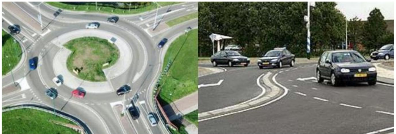
Typical appearance of a Turbo roundabout. Where the new inner lane begins, the idea is not for vehicles to turn into those already in the circulation, which means that U-turns are not always possible in Turbo roundabouts.
